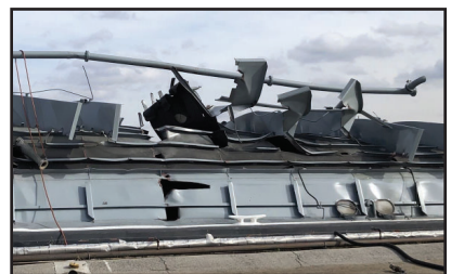
Bent frames & the deformed deck of a red flag barge following an explosion
